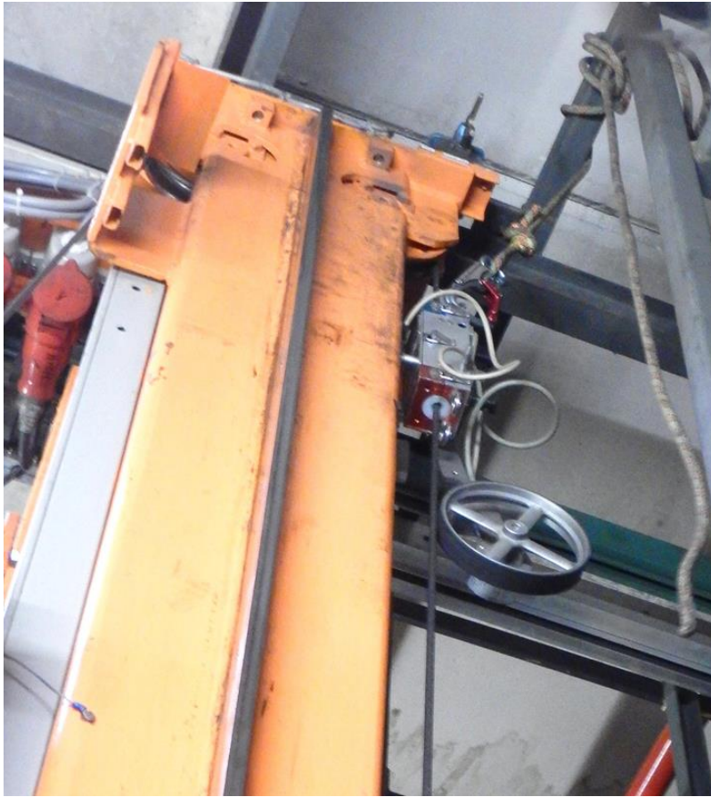
Figure 3: Magnetic inductive rope test on a storage and retrieval machine
